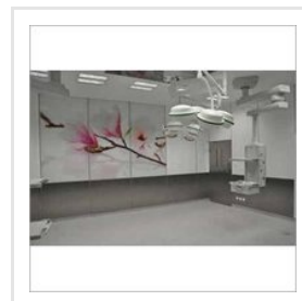
Modular Operation Theatre
